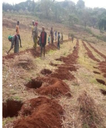
Figure 12. Micro-basin structures of the study area (Source: Field photo, 2023)
