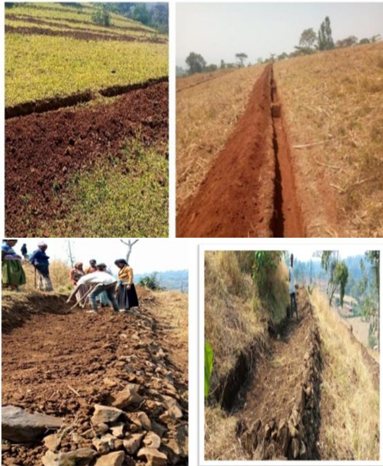
Figure 9. Soil and stone bund structures of the study area (Source: Field photo, 2023)
